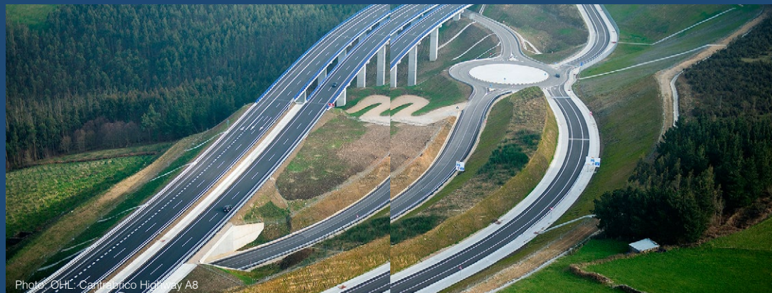
Photo: OHL: Cantabrico Highway A8
